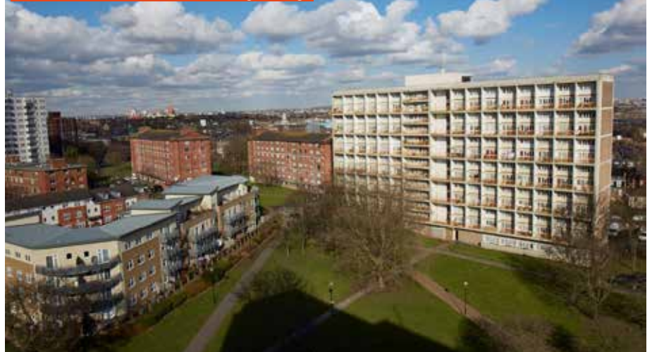
Aerial view of Phase 8.1 and 8.2's existing buildings
